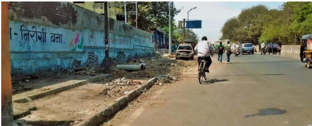
Figure 12: Cyclists and pedestrians forced to use carriage way due to lack of maintenance of cycle tracks and footpaths
