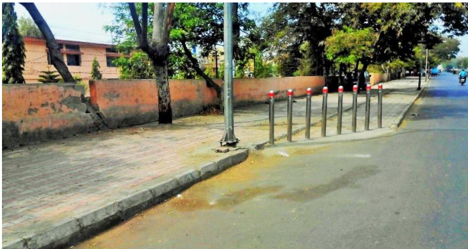
Figure 9: Ill designed cycle lane with bollards breaking the continuity
