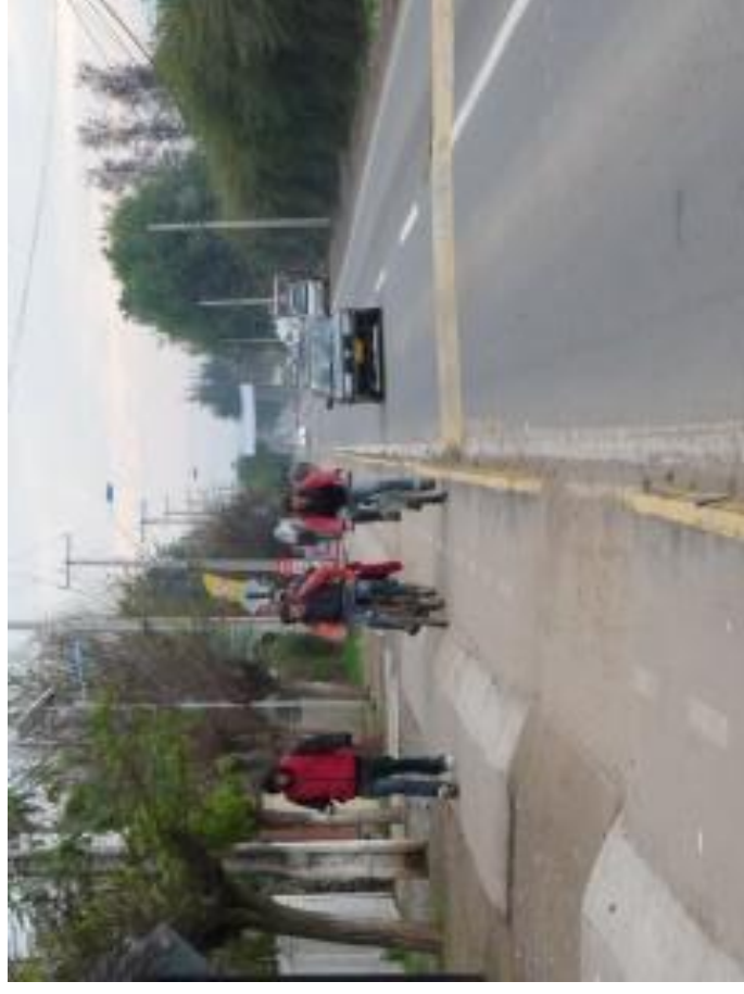
Figure 41: Lack of road safety at road section level. This cycle track is too narrow.
