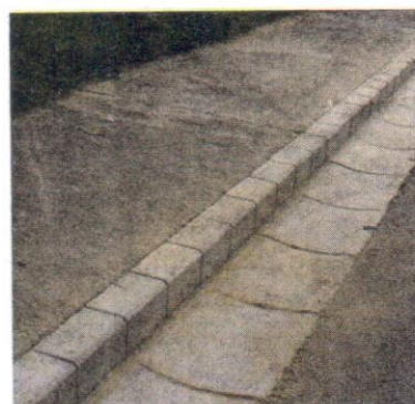
Fig. 27 Kerb Stone Block with Saucer Drain
