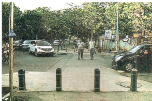
Fig. 12 Footpath continuing at Same Level along Side Street in Chennai
