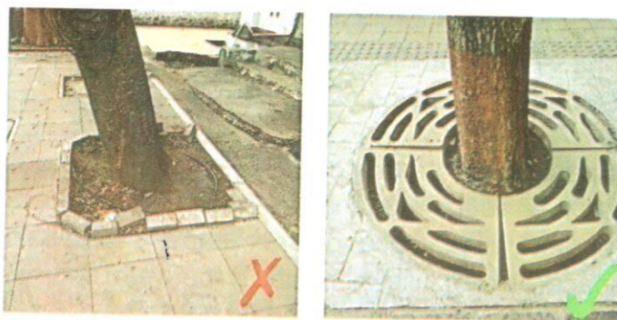
Fig. 54 Tree Grating Detail
