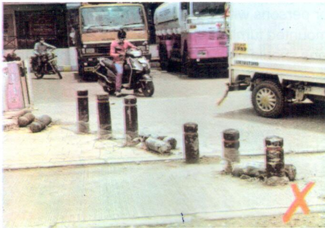
Fig. 35 Broken Bollards due to poor implementation
