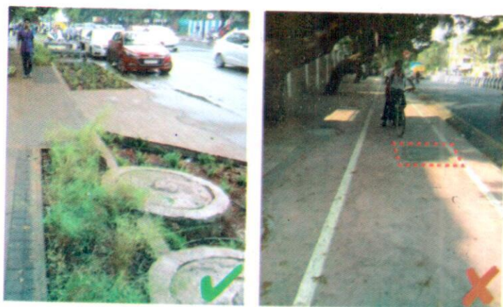
Fig. 44 Service Covers should be located in MUZ
