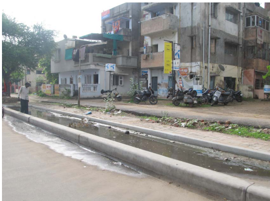
No stormwater run-offs
