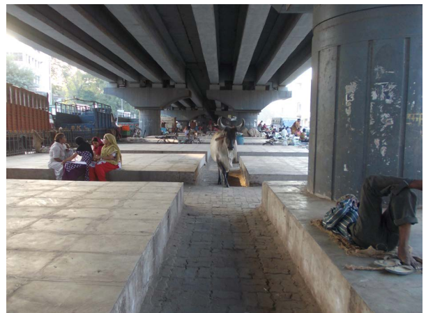
The new platforms - not yet in use
