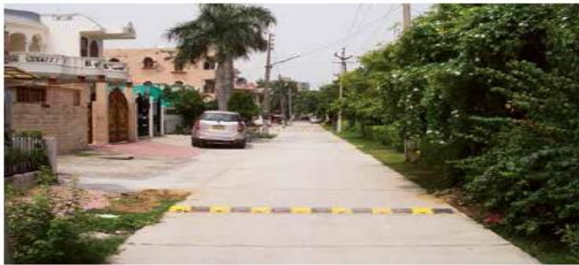
Figure 1: road bump on narrow residential street
