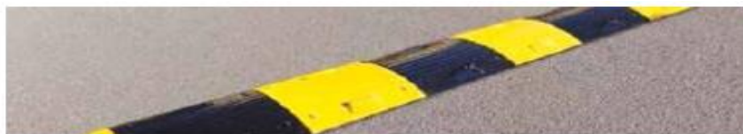
Figure 2: road bump in indian market street
