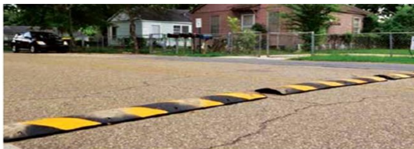
Figure 3: road bump in residential street
