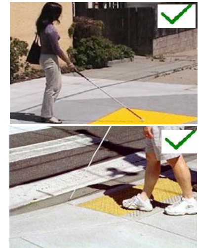
Dot-type block give a warning signal.
