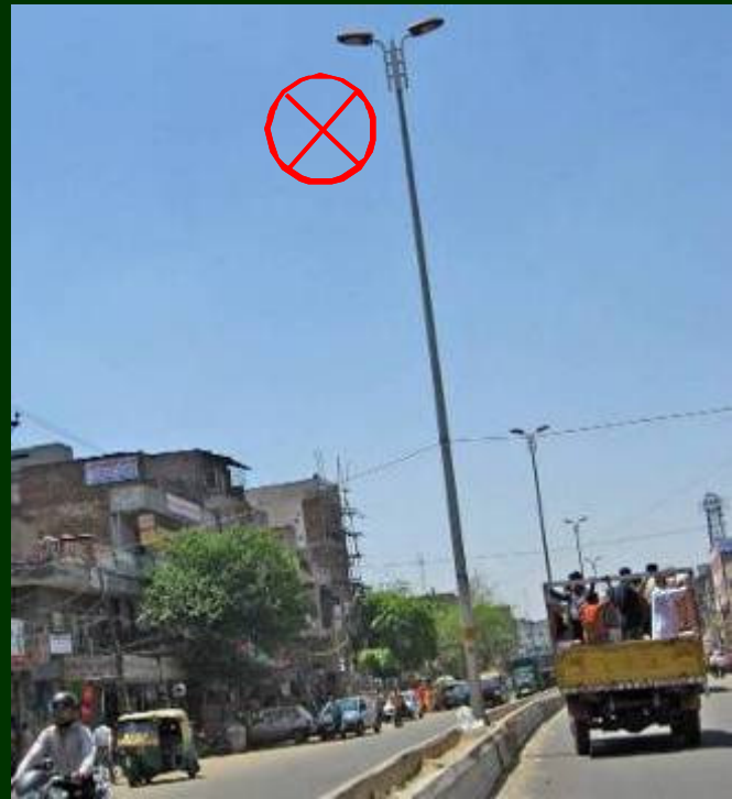
High Mast Lighting is inefficient and ineffective especially in this narrow mixed-use street.
