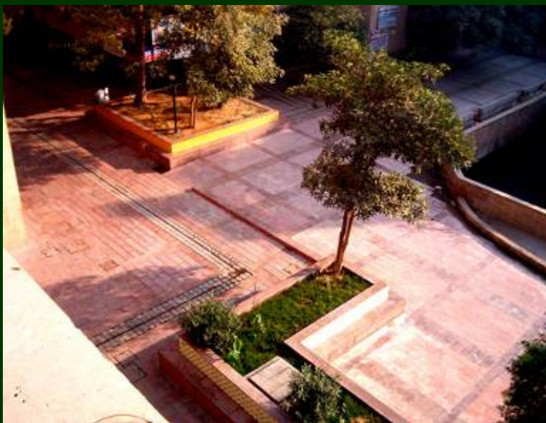
Different colors and textures of Brick and Red Sandstone use to create this warm and well scaled Plaza.
