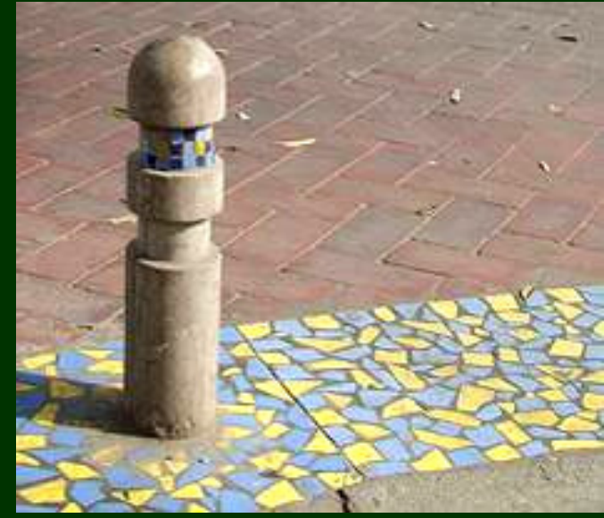
Red tinted PCC Tiles and concrete bollards with glaze Ceramic tile highlights. (BRT Delhi)
