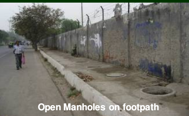
Utilities on Footpath
