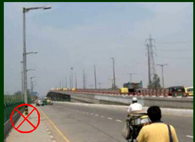
Light poles placed on the walkway so pedestrians are forced on to the road.
