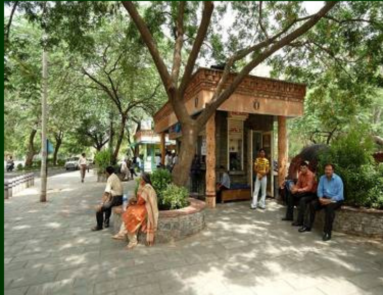
Paving in Rough Kotah stone. Seats in stone masonry. Kiosk columns clad in ceramic mosaic. (Vikas Sadan, Delhi)
