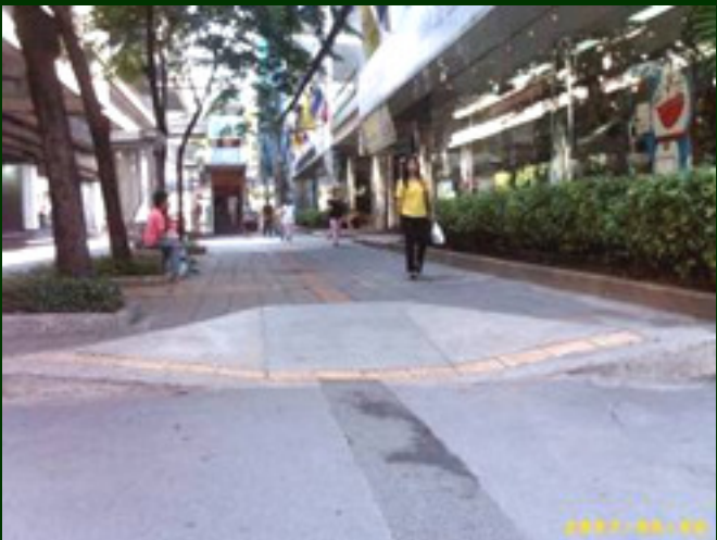
Kerbed Ramp with Tactile Paving
