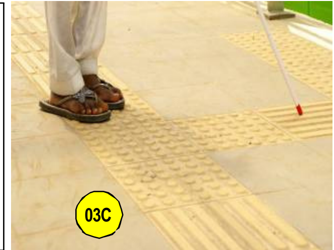
Engineering configuration of floor tactile tiles
