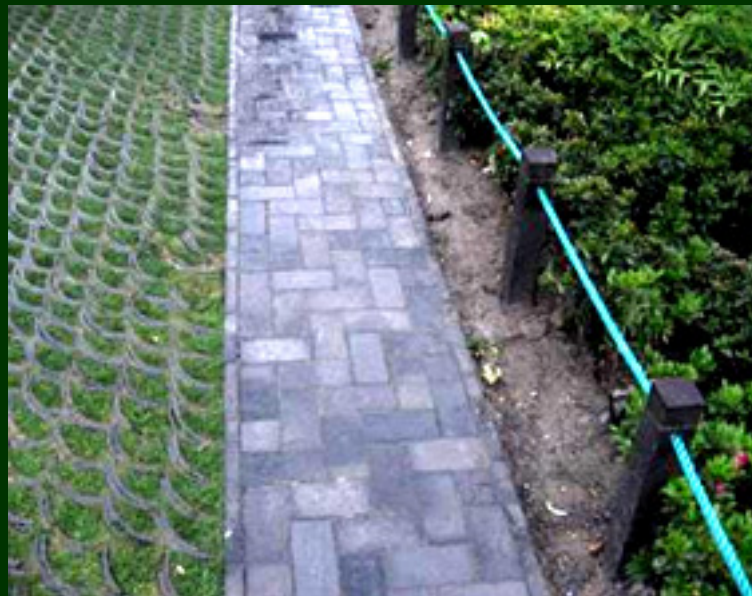
Permeable grass pavers use in sloped seating area with walkway in rough finished stone pavers. (Shanghai)
