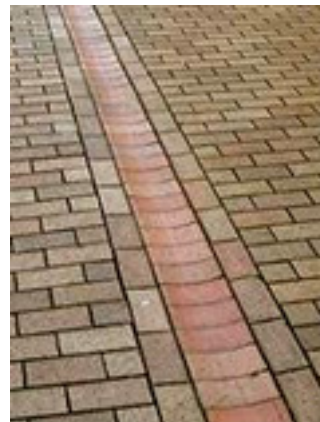
Brick Drainage Channel in Walkway
