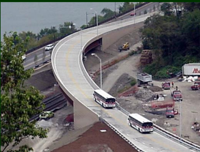
Dedicated Bus ramp
