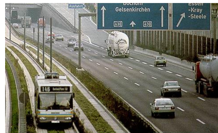
Montage of Guided busways in Essen, Germany
