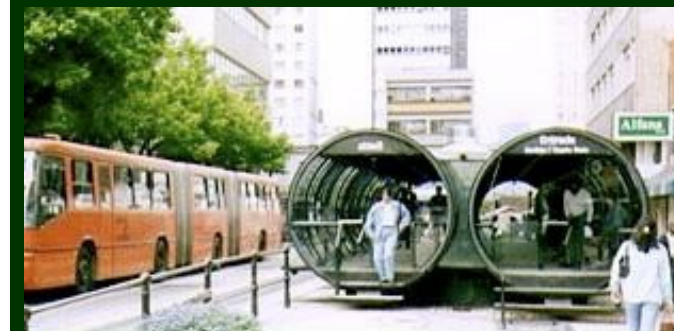
Distinct BRT stations at Curitiba, Brazil
