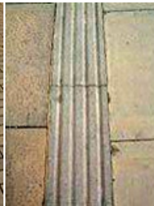
Fluted Drainage Channel in Walkway
