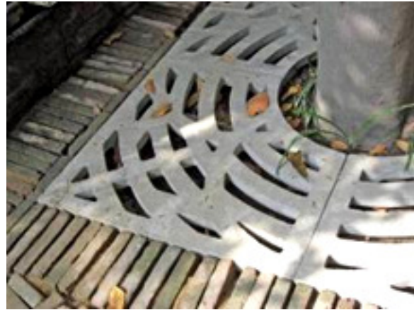
Sample Detail of Precast Cement Concrete Tree Grating. Source: Pradeep Sachdeva Design Associates, Nov 2009
