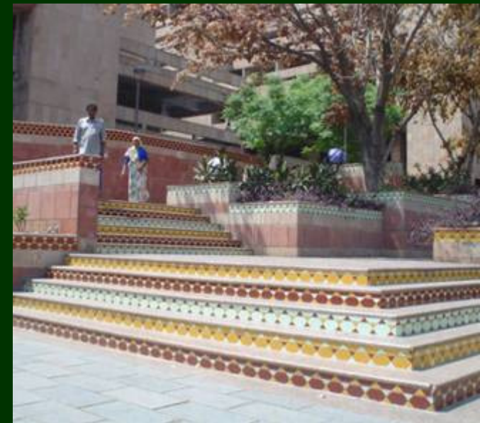
Ceramic Tiles use on vertical surfaces and risers of steps to add color (Bikaji Cama Place, Delhi)
