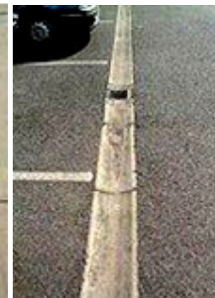
Concrete Drainage Channel in Asphalt Pavement
