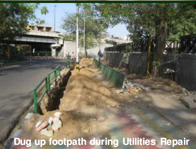
Open Manholes on footpath
