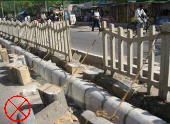
Median fences totally inappropriate, especially on a residential, mixed-use, slow traffic street.
