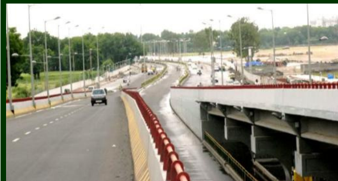
Treatment of existing flyover at Ahmedabad.
