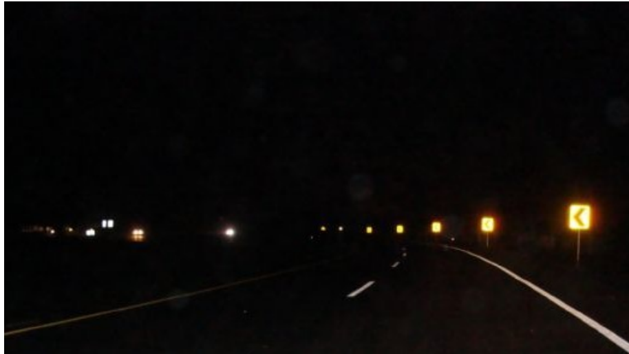
Figure A.10: Example of signs and/or line marking Retroreflective chevron signs providing visibility at night. (Source: iRAP)
