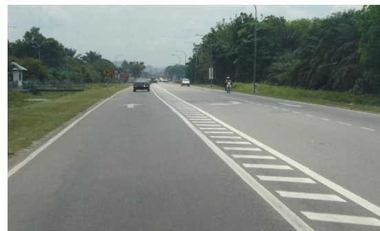
Figure A.5: Painted median/central hatching. (Source: iRAP)
