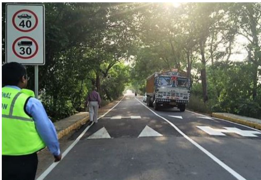
Figure A.17: Gateway treatment between a high speed and low speed environment (Source: World Bank)
