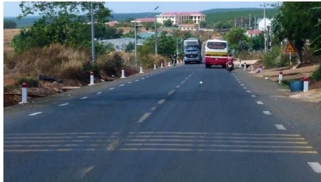
Figure A.12: Example of transverse ATLM Transverse rumble strips in Vietnam. (Source: World Bank)
