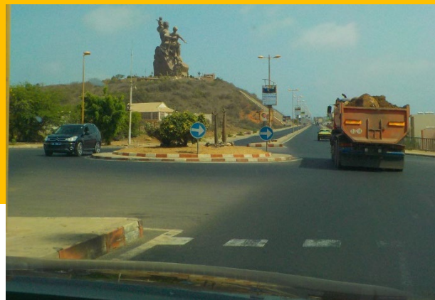
Poor deflection (Source: GRSF)
