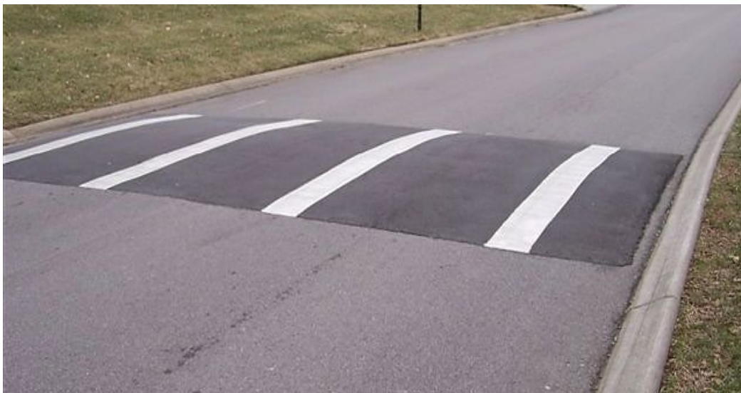
Figure A.15: Traffic calming/Speed Hump (Source: NACTO)
