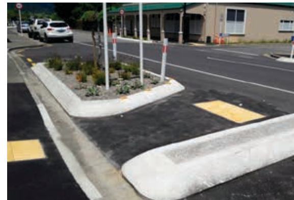
Source: New Zealand Transport Agency (© J Ward).
