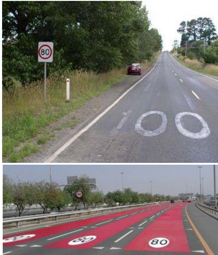
Figure 51: Lane Wise Speed Markings
