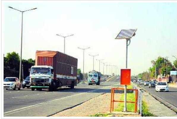
Figure 44: Telephone booth near carriageway for emergency
