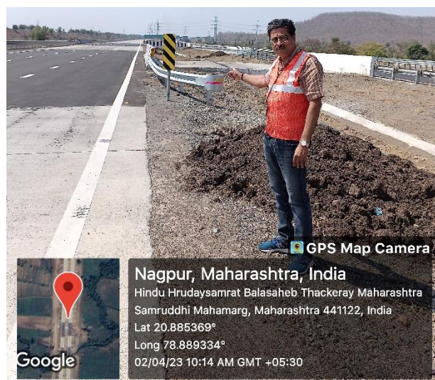
Figure 59: Object Hazard Markers were placed wrongly, observed during road inventory survey
