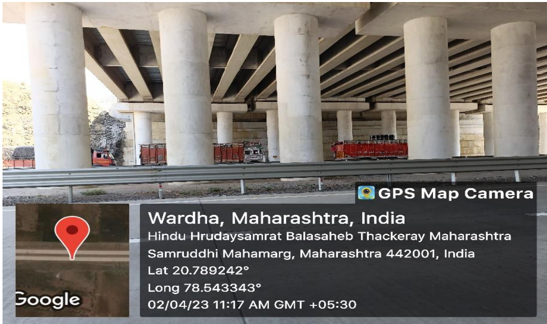
Figure 56: Trucks were found parked under the overpass during road inventory survey.
